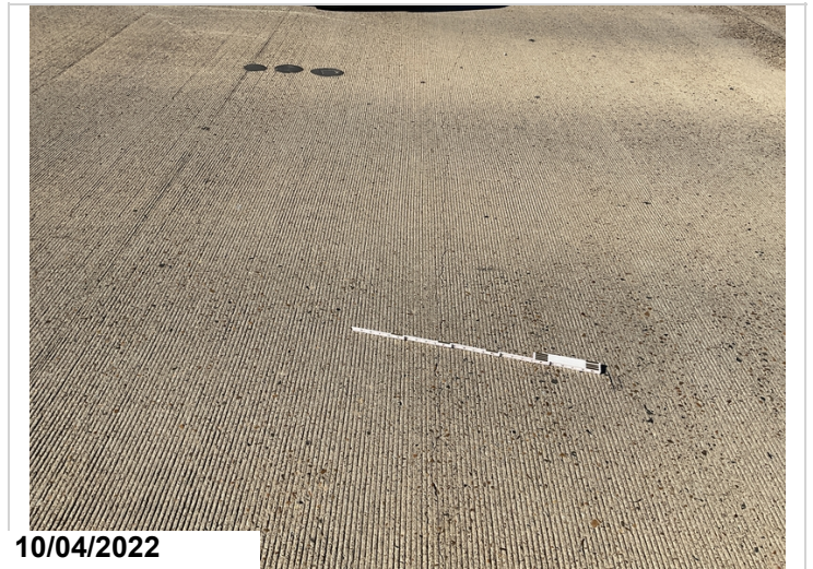
Span 5: unsealed transverse cracks. Common to all spans.
