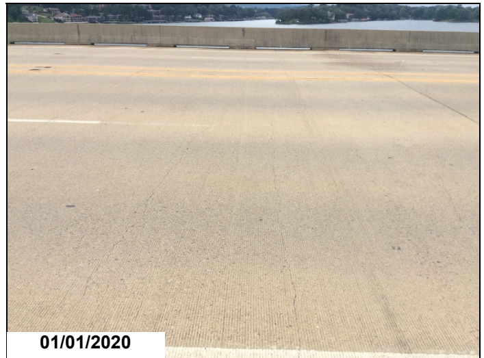
Span 5 transverse cracks.
