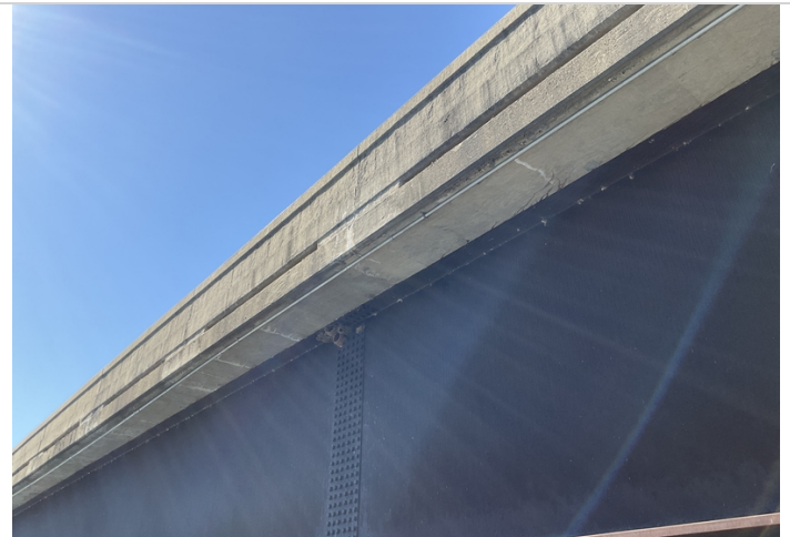
Span 5: Overhang has transverse cracking with efflorescence staining.
