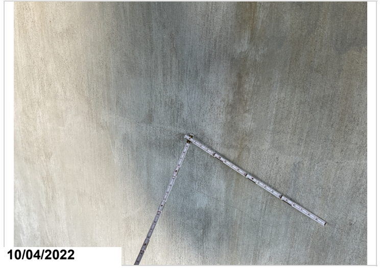
Backside of bent 3: Vertical and diagonal cracking up to 0.020".
