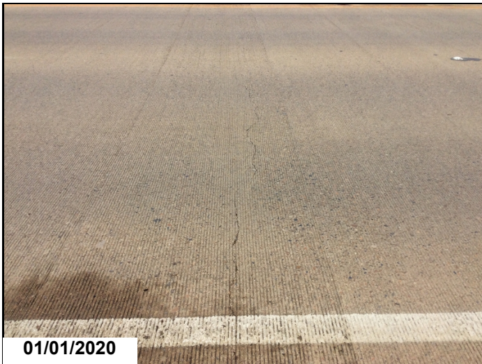
Transverse crack in span 2.
