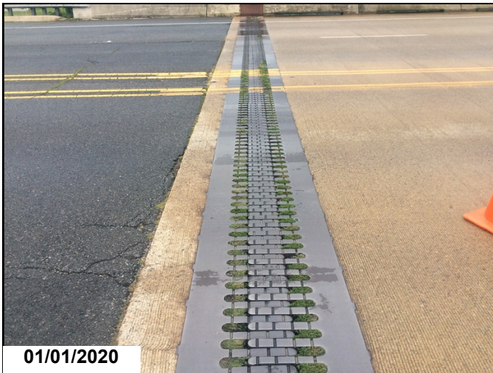
Bent 8 joint is full of debris.
